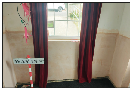
and on the right is the re-plastered foyer
