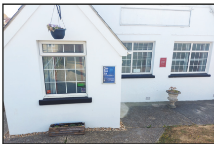
On the left is the freshly painted front elevation
